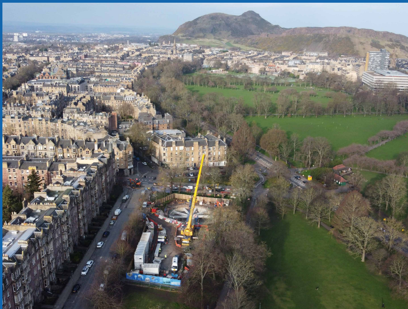
Work being carried out in Edinburgh's Marchmont area to reduce flooding
